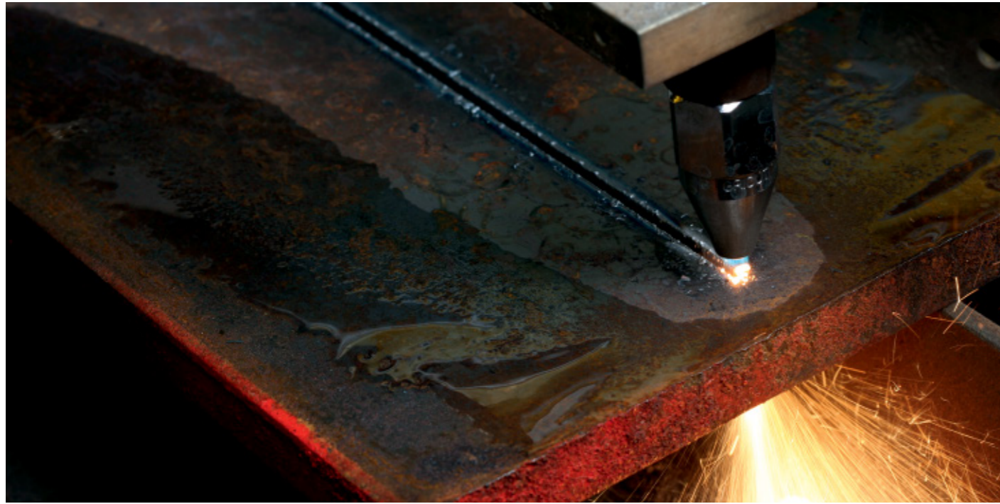
Water puddles formed on a cool plate during oxy-propane cutting. Moisture leads to corrosion and causes problems when preheating, brazing or welding.
