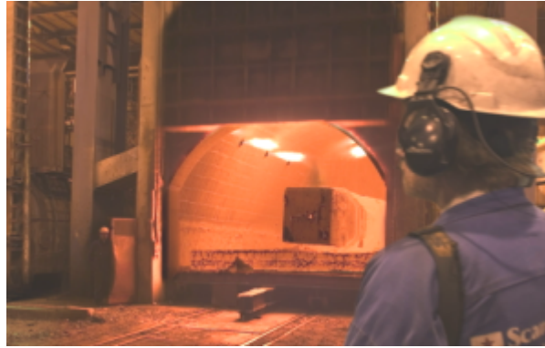
Figure 3, Flameless oxyfuel employed in car bottom furnace for reheating prior to forging at Scana, Sweden. It has resulted in more uniform heating and reduced emissions of NO x .
