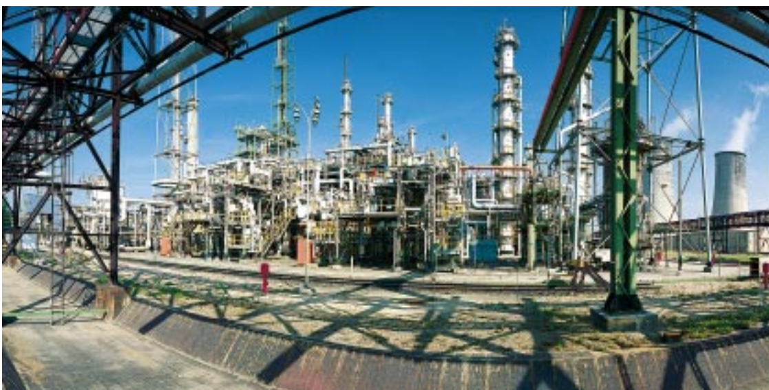
Left: Production of syn- thesis gas and methanol from oil refining residues
