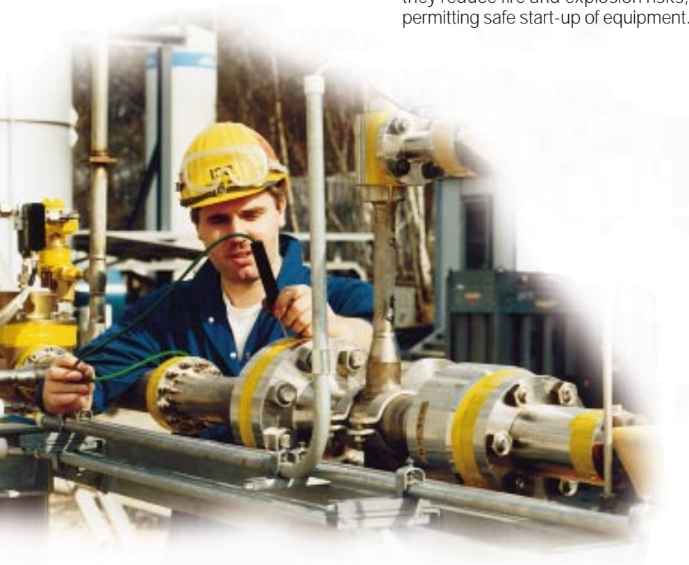
Leak test on piping assembly for hydrogen plant
